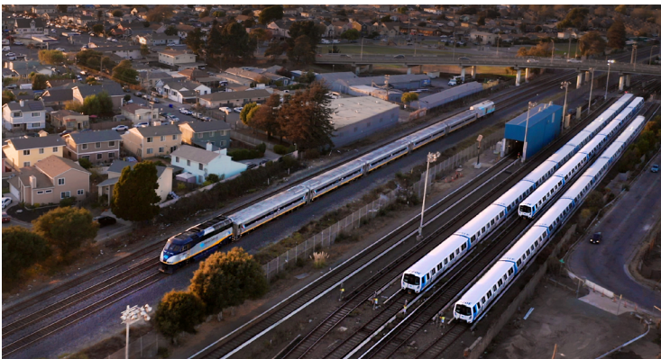
Link21 will create better connections between Northern California intercity train services and BART.
